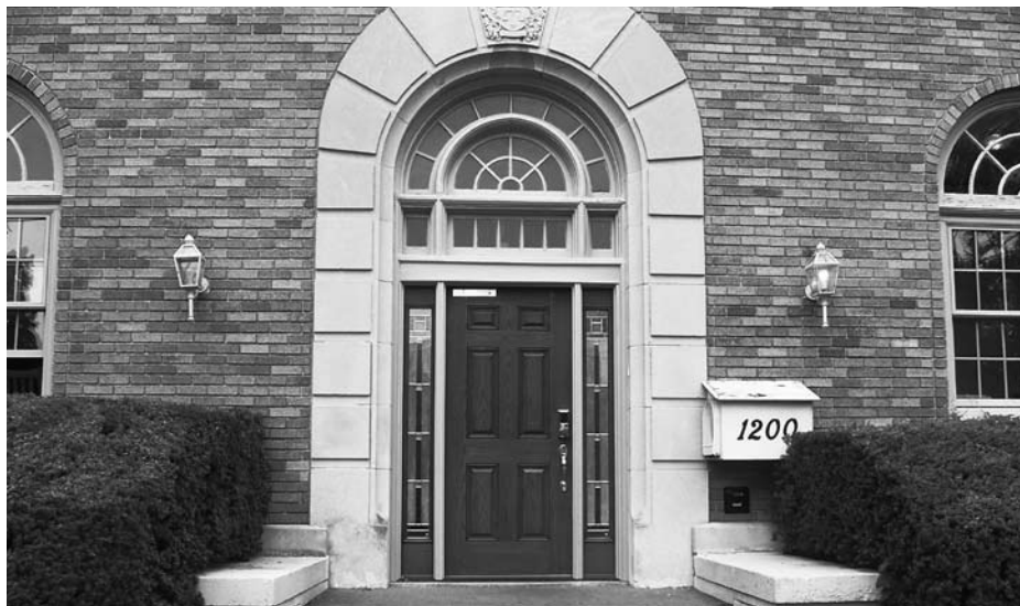
A new Ballantine Street door adds elegance and privacy to the west entrance of the DU house.
